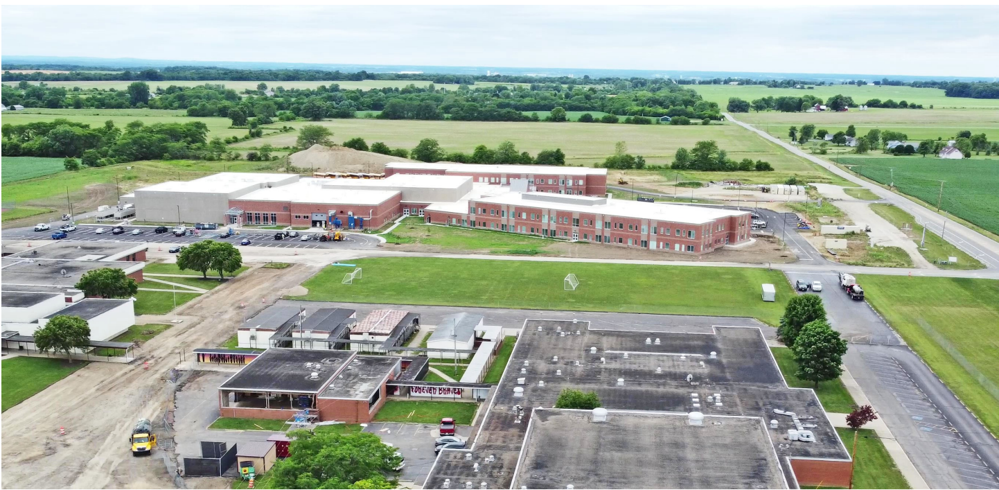
New school under construction
